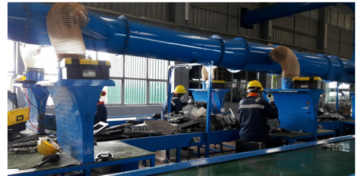
Enviroserve Rwanda, Dismantling Stations at their facility
